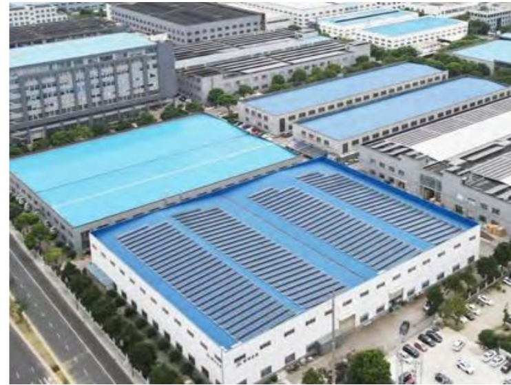
8WM On-Grid Solar System
